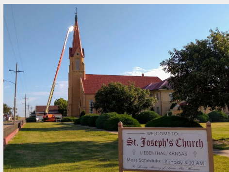
The camera captures a reflection as workers replace copper on the steeple of St. Joseph Church in Liebenenthal in 2019.
